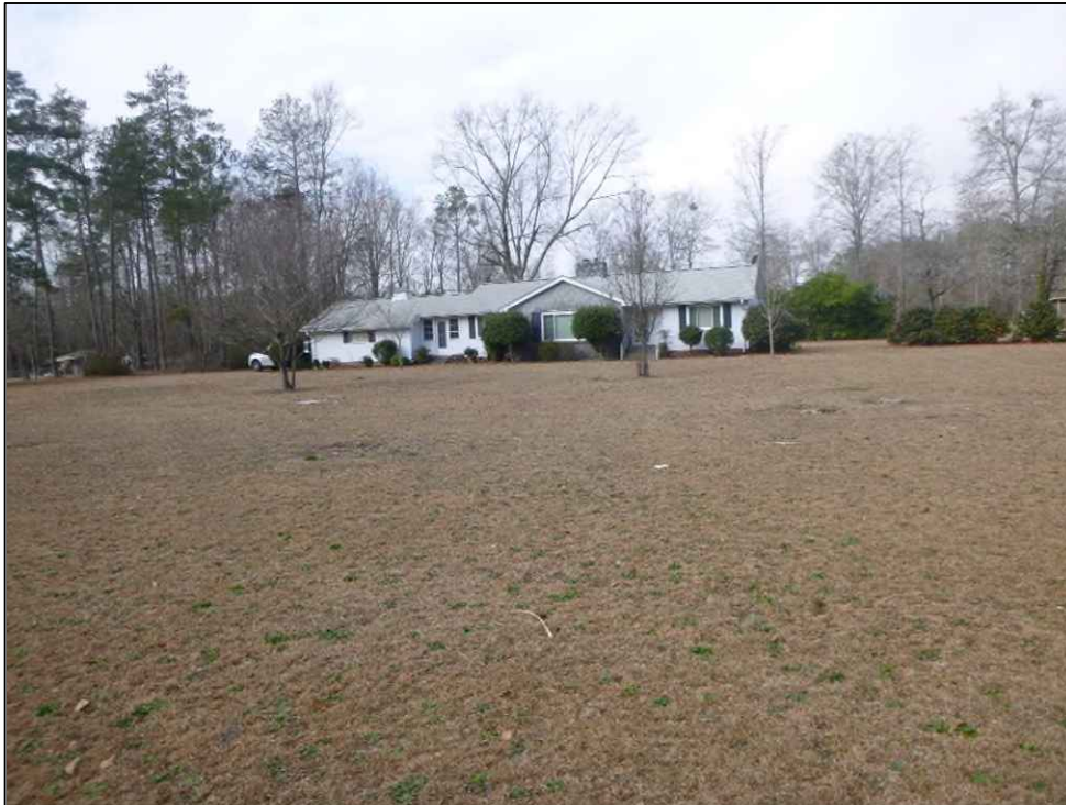
Figure 5.14. SHPO Survey Number 8727, facing southwest.
