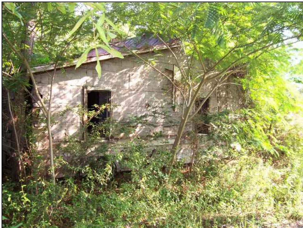
Figure 45. House associated with Site 38RD1299, facing north.
