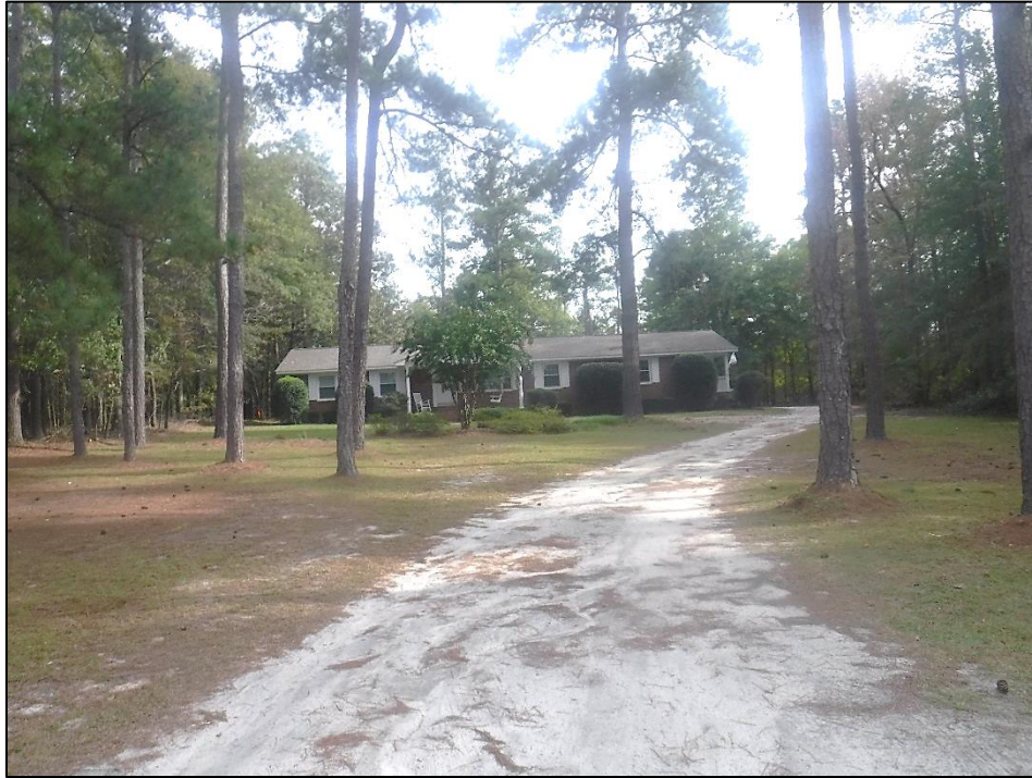
Figure 5.42. Structure 7621, facing southeast.
