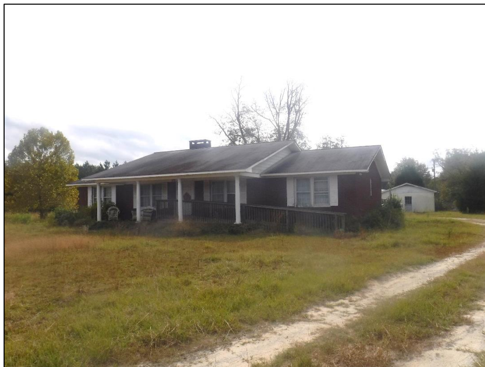
Figure 5.37. Structure 7619, facing southeast.
