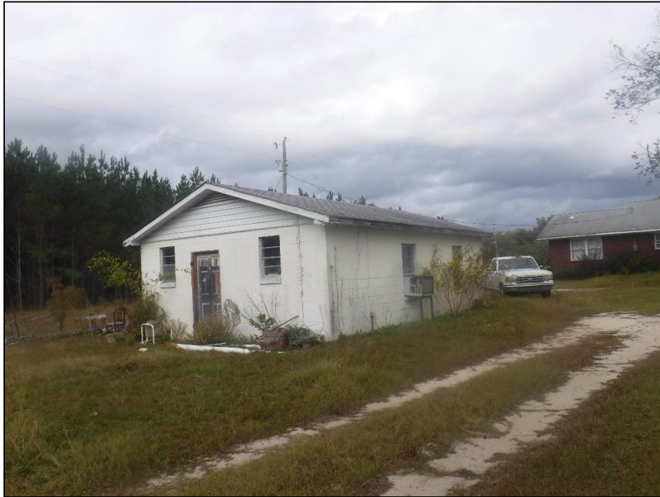
Figure 5.38. Structure 7619.1, concrete block garage, facing northwest.
