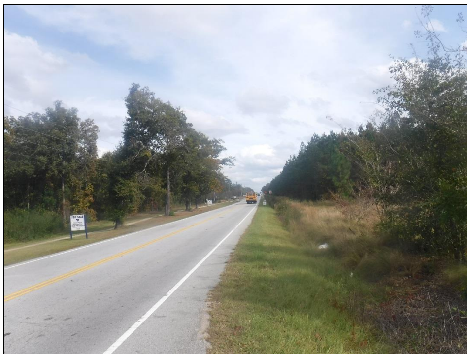
Figure 5.45. Blythewood Road (7623), facing east.
