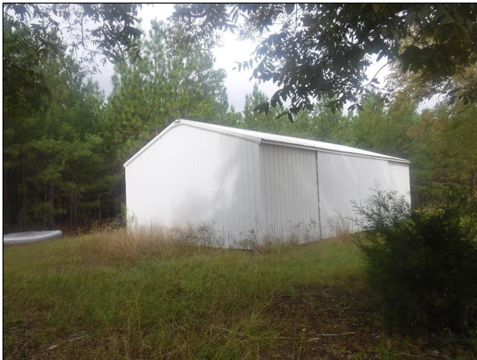
Figure 5.39. Structure 7619.2, modern storage shed, facing northwest.
