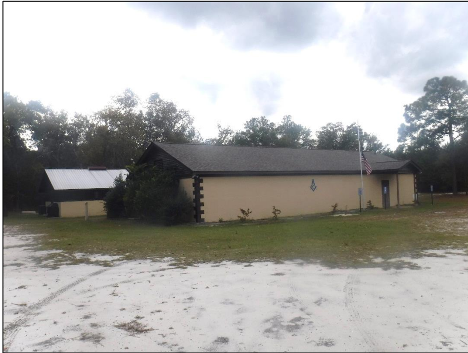
Figure 5.41. Structure 7620, facing southwest.
