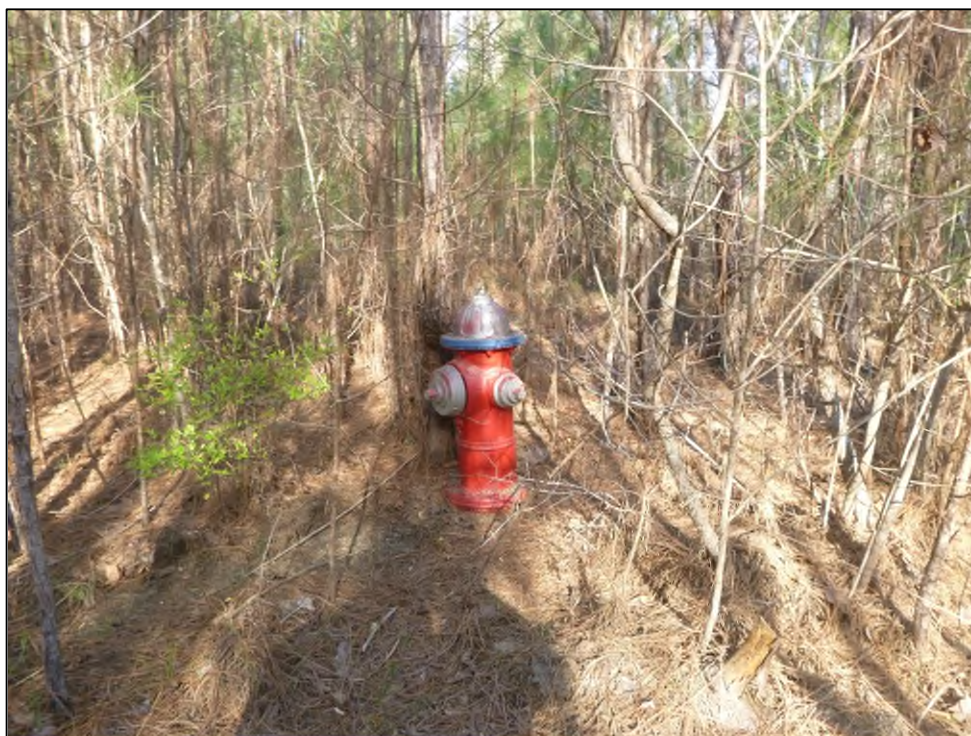
Figure 5.3. Buried utility in the project area, facing northwest.
